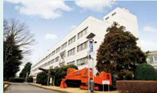
Tsuchiura Works East Building and the Hitachi UH03 hydraulic excavator, which is included in the list of Japan's Mechanical Engineering Heritage.
