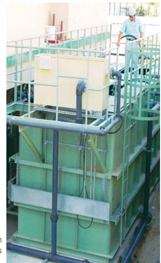
A PERSEUS system installed at a construction workers' housing complex in Dubai processes wastewater for about 1,500 people.
