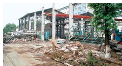
(Top) Hitachi Construction Machinery excavators, important for earthquake recovery (Bottom) Earthquake damage at Dongfang Electric Corporation's Hanwang plant
