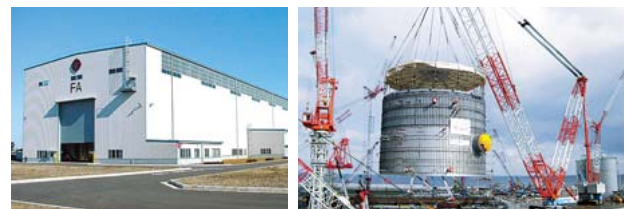
(Left) Module assembly factory (Hitachi Works, Hitachi GE Nuclear Energy) (Right) Nuclear reactor containment vessel being lifted into Unit No. 3 at Chugoku Electric Power Company's Shimane Nuclear Power Station in Japan
