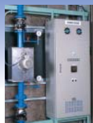
Energy back system Integrated generator and hydraulic turbine
