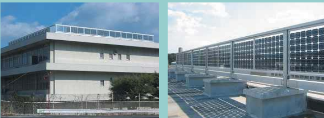
Testing out solar power generation in the form of a rooftop fence on a building located in Hitachi works
