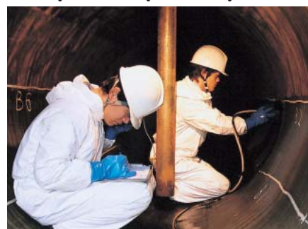
Inspecting for corrosion in an underground water tank
