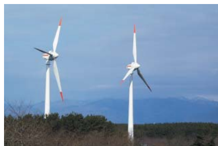
Two 600 kW wind power generators erected at the Noshiro Ochiai Wind Power Plant.
